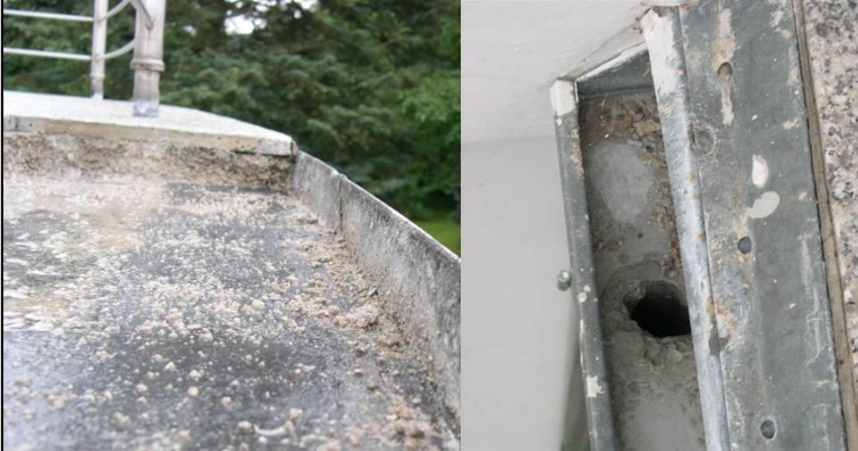
AUSGESCHWEMMTER BETON KORROSIONSGEFAHR
