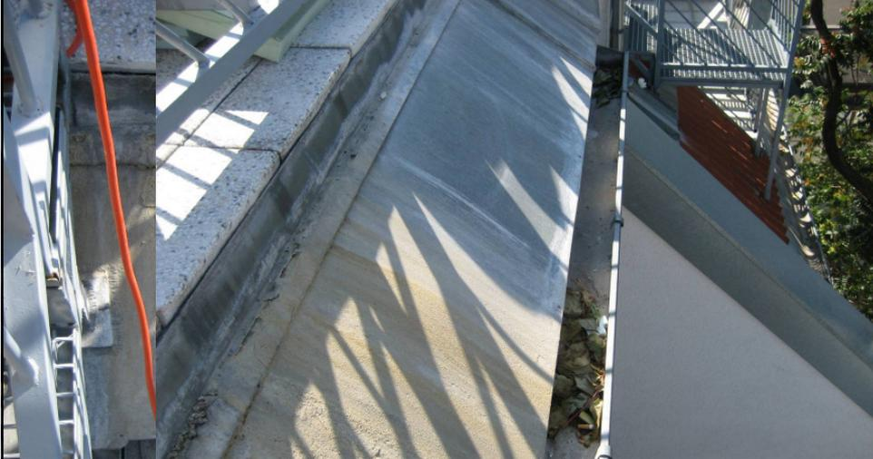
**AUSGESCHWEMMTER BETON KORROSIONSGEFAHR**
