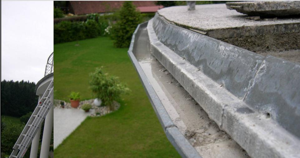
**AUSGESCHWEMMTER BETON KORROSIONSGEFAHR**
